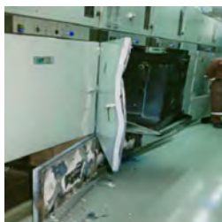
Representative views of switchgear damaged or destroyed by the effects of an arc fault.
